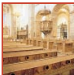
In Ribe Cathedral Logia has installed an audio system including 144 pews with built-in loudspeakers, hand-crafted in oak. When a person sits down sensors automatically activate the loudspeaker.
